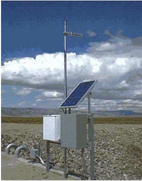
TYPICAL SOLAR RTU/RADIO
